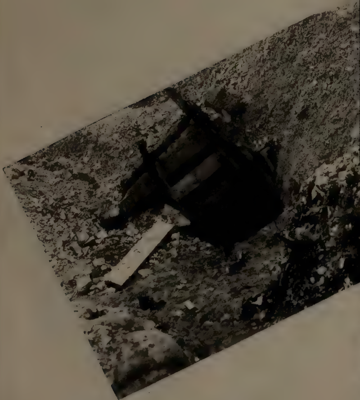
1. Looking out of the famous Bismark Tunnel, which was driven thru the Hill by the Germans. It is about seven ft. in height and wide enough for four men abreast. It contained a perfect Ventilating and Drainage System. At intervals there were large Chambers built off from the sides.
